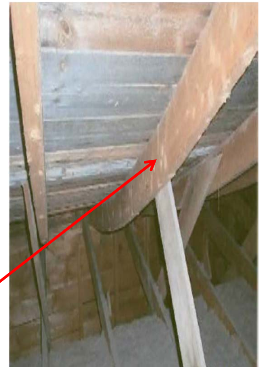
Broken wood truss
